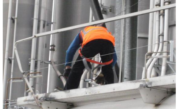
Harness not fitted correctly
